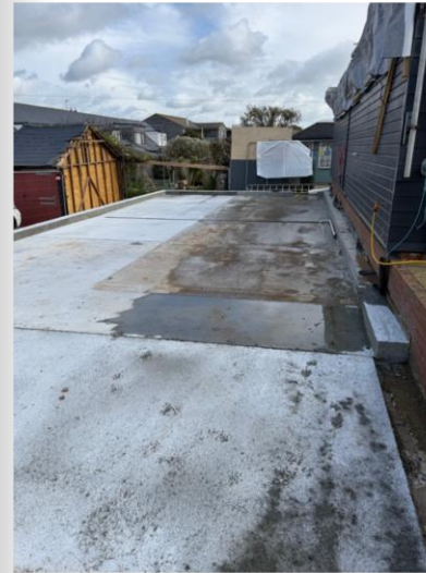
Ground works completed.
